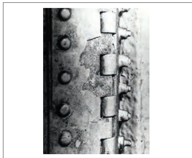
Figure 3-17. Piano Hinge Lugs
