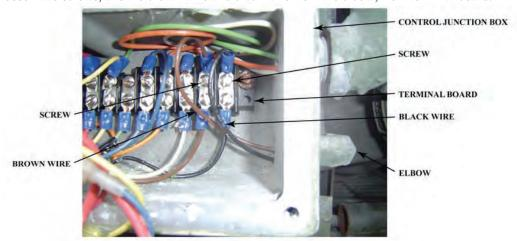
4. Loosen nut and remove conduit tube from elbow. Pull brown wire and black wire out through elbow. Remove elbow from control junction box.
