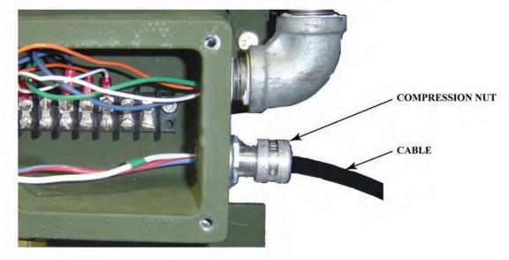
3. Install red and blue wire on terminal block, matched to existing red and blue wire. Install white wire with green tape on terminal block, matched to existing green wire. Other wires shown removed for clarity.
