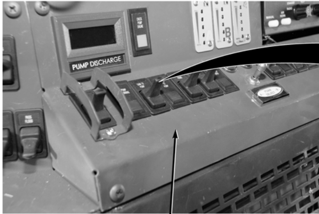
CAB PUMP CONTROL PANEL
