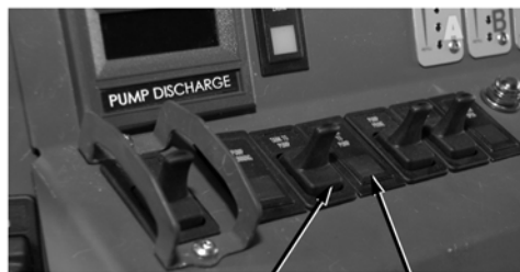
TANK TO PUMP SWITCH TANK TO PUMP INDICATOR
