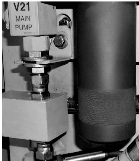
Figure 3-41. Valve Components Shown Installed in Support Bracket
