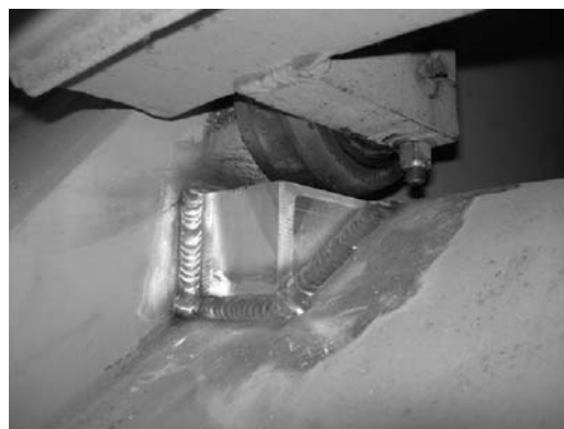
Figure B-4. Wheel Support Wedge Welded in Position
